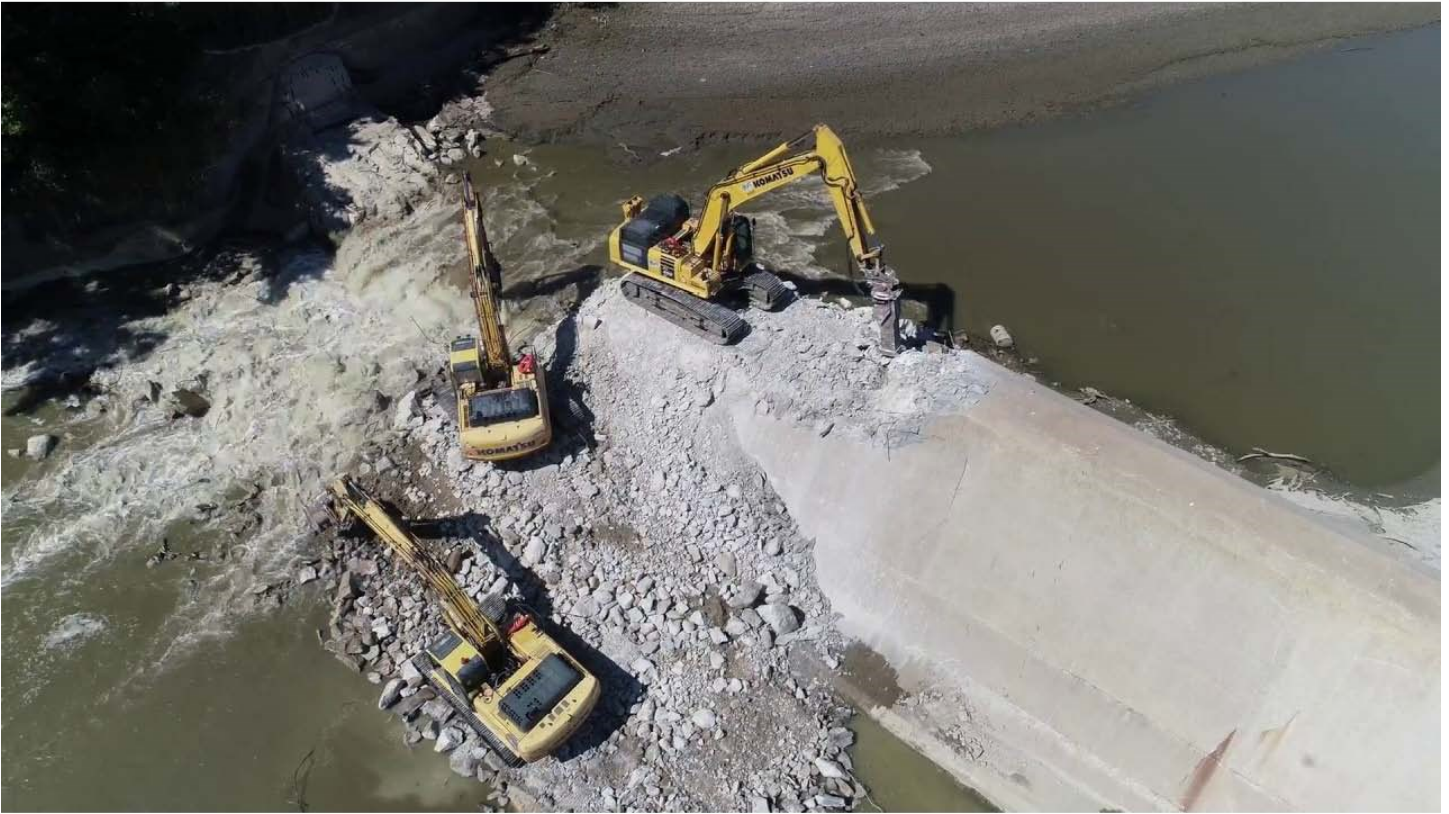
Removal of Spillway (Ballville Dam, Fremont, OH)
